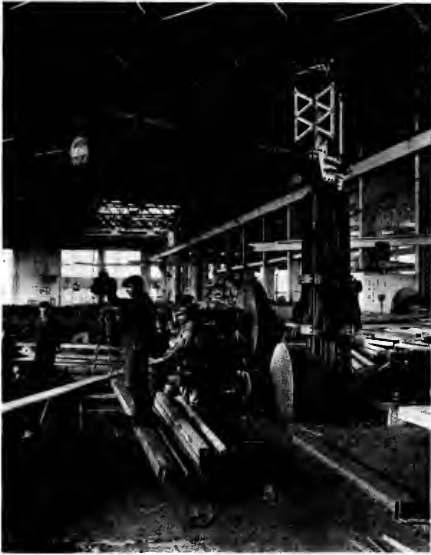
Fig. 7. A 3-ton, 2 double part reave, electric hoist, mounted on a self-supporting bracket crane. The machine shown is a heavy punch used for punching deck beams and ship frames.
